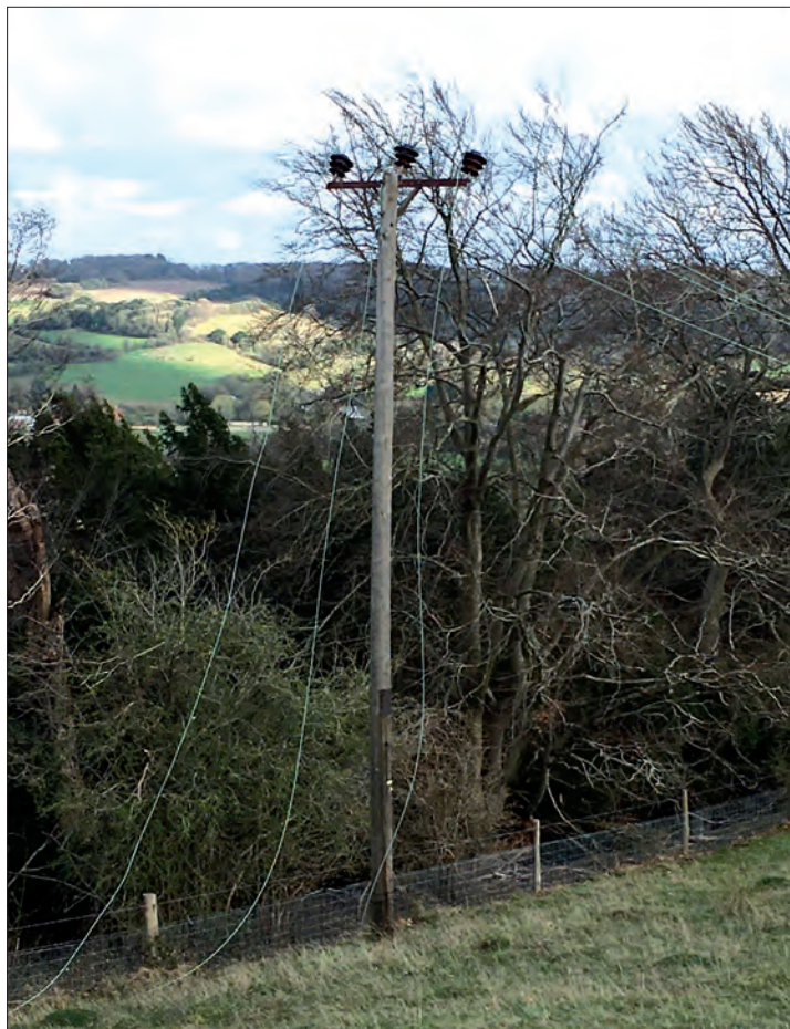
Broken electricity cable due to the poles to the left falling.
